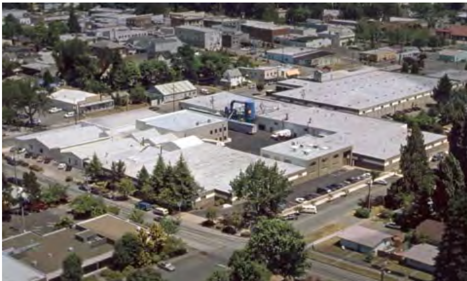
The Woodfold manufacturing facility at Forest Grove, Oregon.
